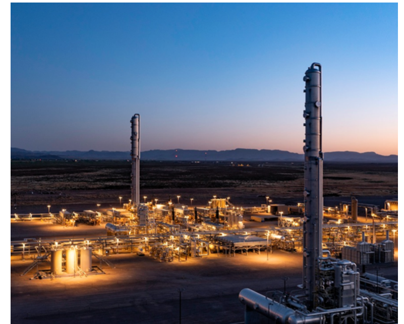
Diamond Cryogenic Processing Plant designed with Dark Skies-Friendly Lighting practices. Light pollution has harmful effects on the natural cycles of plants and wildlife. In collaboration with Texan by Nature, their Recommended Lighting Practices were implemented during construction of the Diamond Plant and other facilities. These conservation efforts include using warm-colored bulbs and installing downward-facing light fixtures directed away from the sky.
